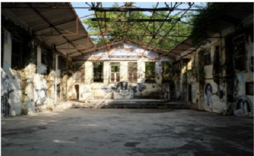
Damaged sheet roof of the yoga hall
